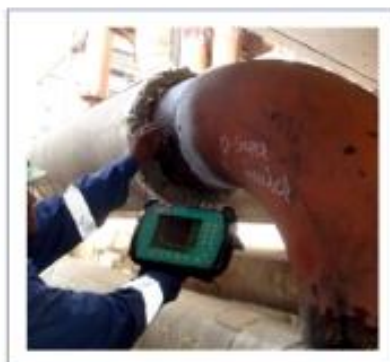
Ultrasonic Testing of De SuperHeater Pipe
