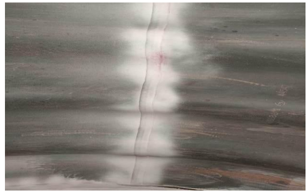
Photo 11: No surface indication observed in all weld joints of vessel in Liquid Penetration Testing.
