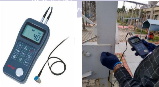
Ultrasonic thickness gauge survey at Leg of Column
