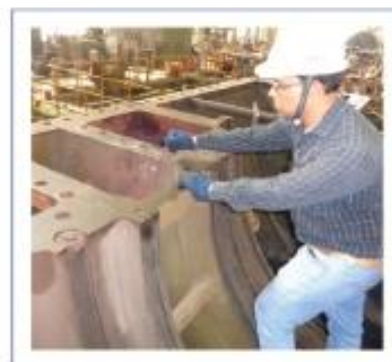
Visual Inspection of LP Casing
