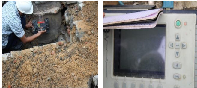
Testing of cover by a meter
